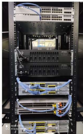
Site Photo (Front View)
